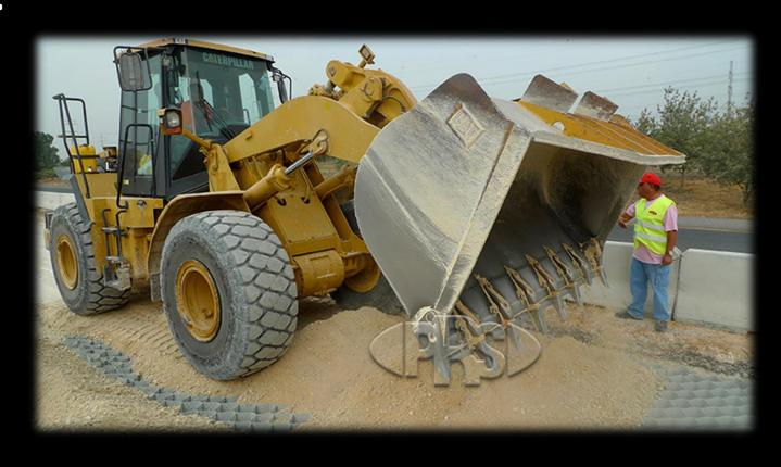
AECON tested PRS Neoloy Tough-Cells in several pavement sections.
