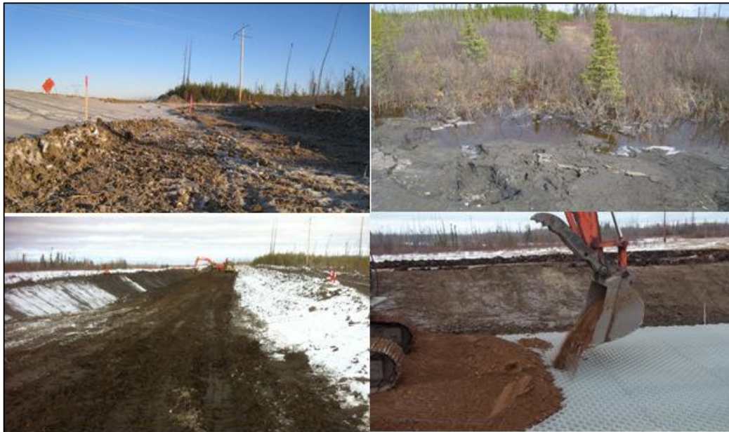
Figure 4: Construction (top left: Frozen muskeg, top right: Water at Ground Level, bottom left: before Installing Neoloy, bottom right: Installed Neoloy)
