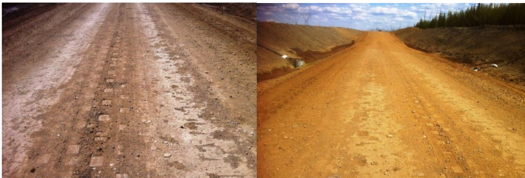
Figure 6: Causeway Surface after 3 Months of Use
