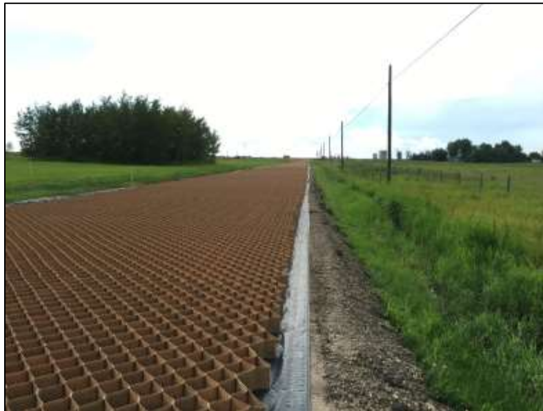
Figure 1 Stretched NPA Geocells ready to be infilled with gravel
