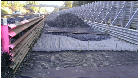
Fig. 7 Installation of the geocell material to build geocell reinforced track
