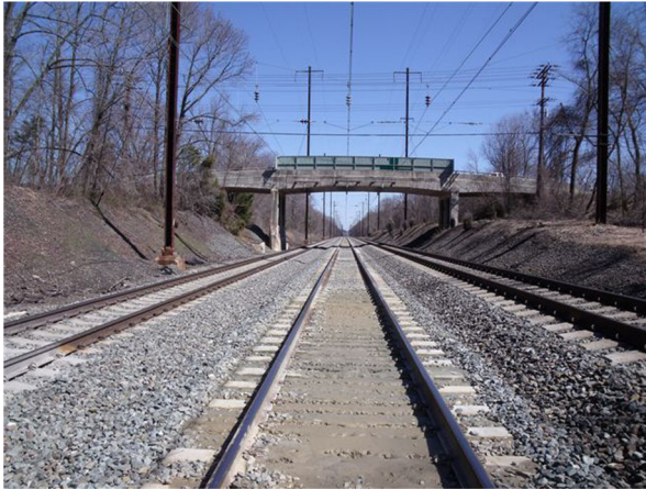
Fig. 1 Fouling and mud spots at Oakington Road, 2010
