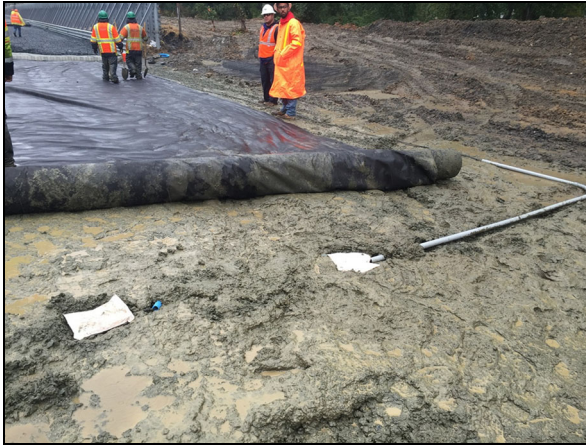
Fig. 6 Pressure cell installation in no geocell zone
