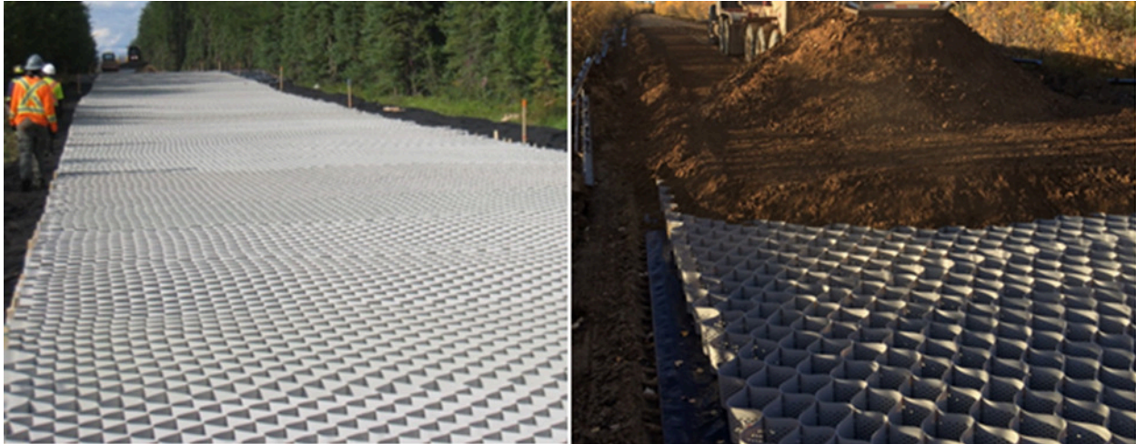
Figure 1: Geocells stretched and being infilled
