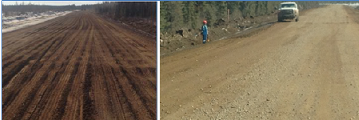
Figure 3: Driving condition on C-road a) before and b) one year after construction
