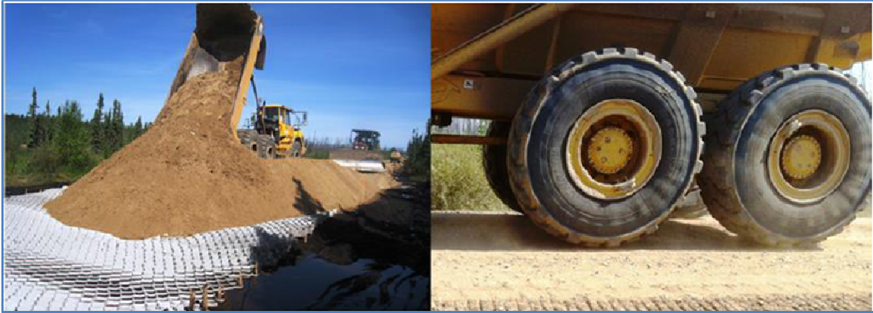
Figure 2: P-3 connector a) during construction and b) during the heavy traffic operation
