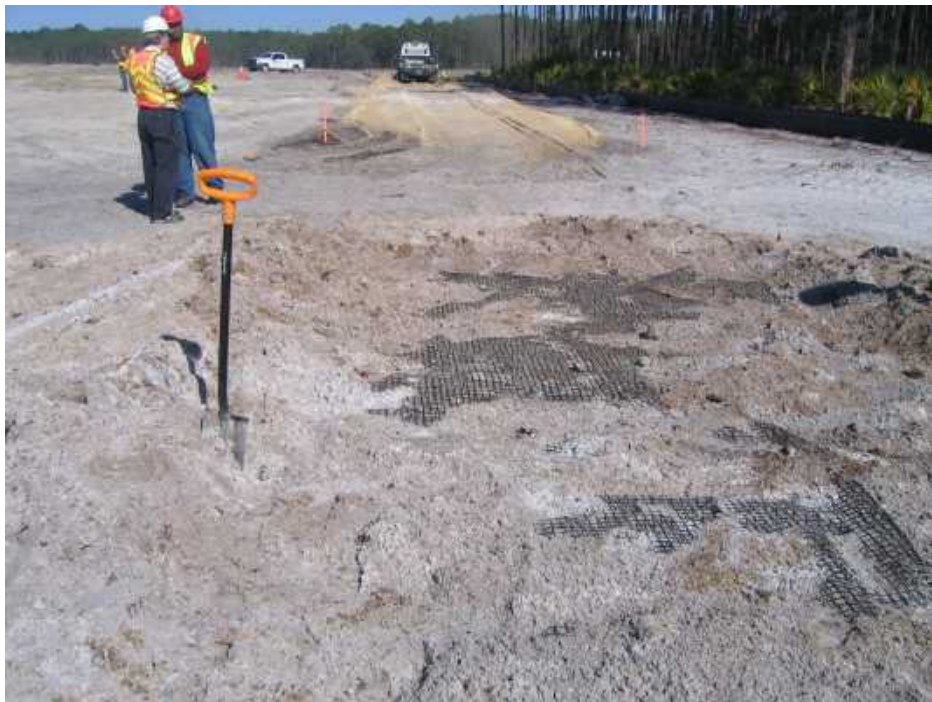
Figure 69. Installation of BX geogrid on TB2
