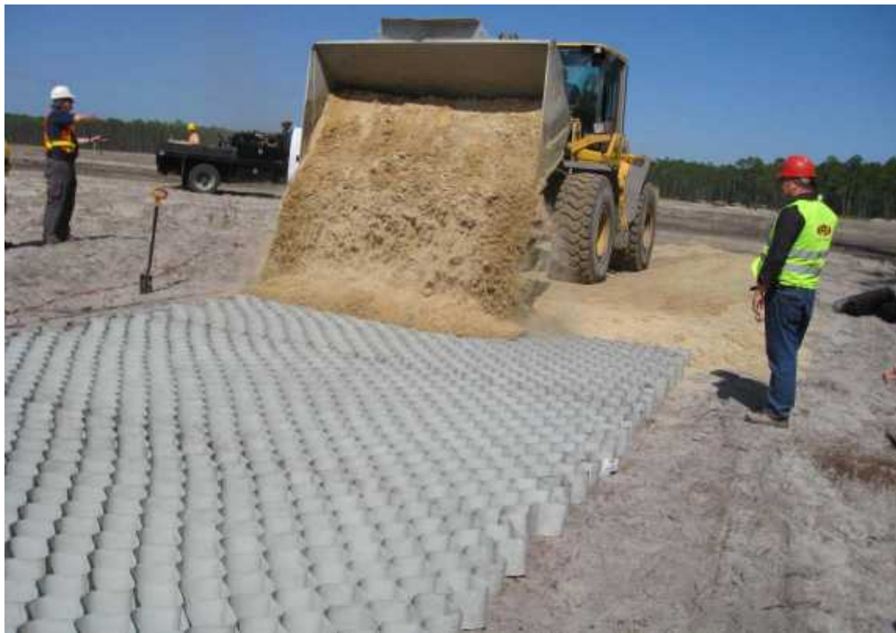
Figure 7. Placement of infill material into geocells
