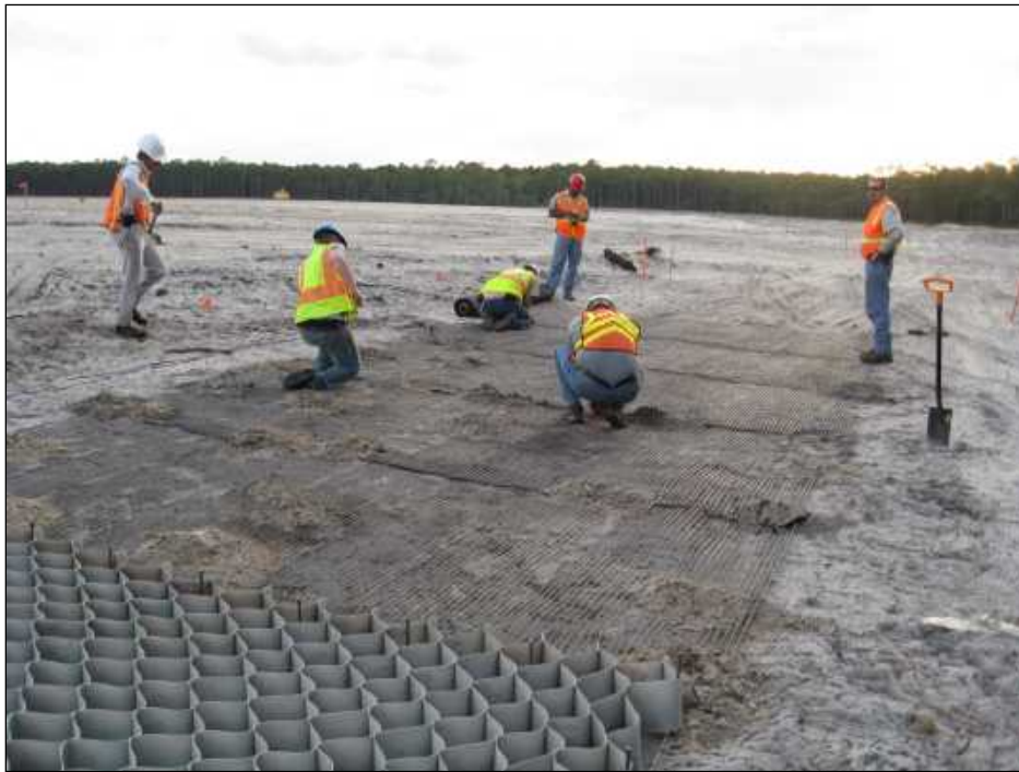
Figure 22. Biaxial (BX) geogrid placed on the sand base layer – TB1
