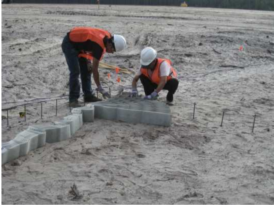
Figure 23. Rebars or pegs installed in transverse and wheel directions to aid in stretching the geocells – TB1
