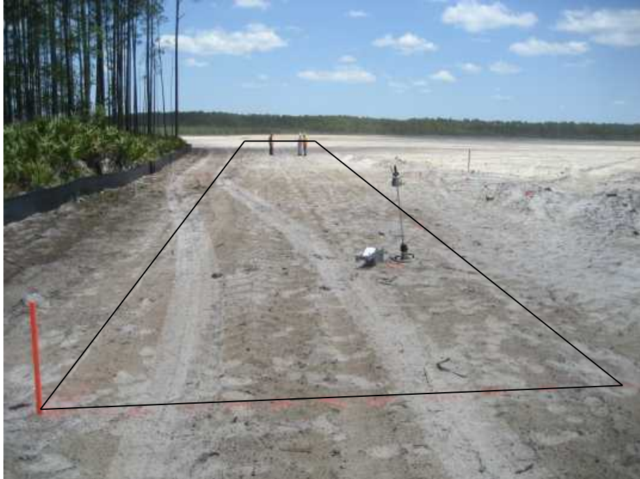
Figure 19. Existing sand base layer – TB1
