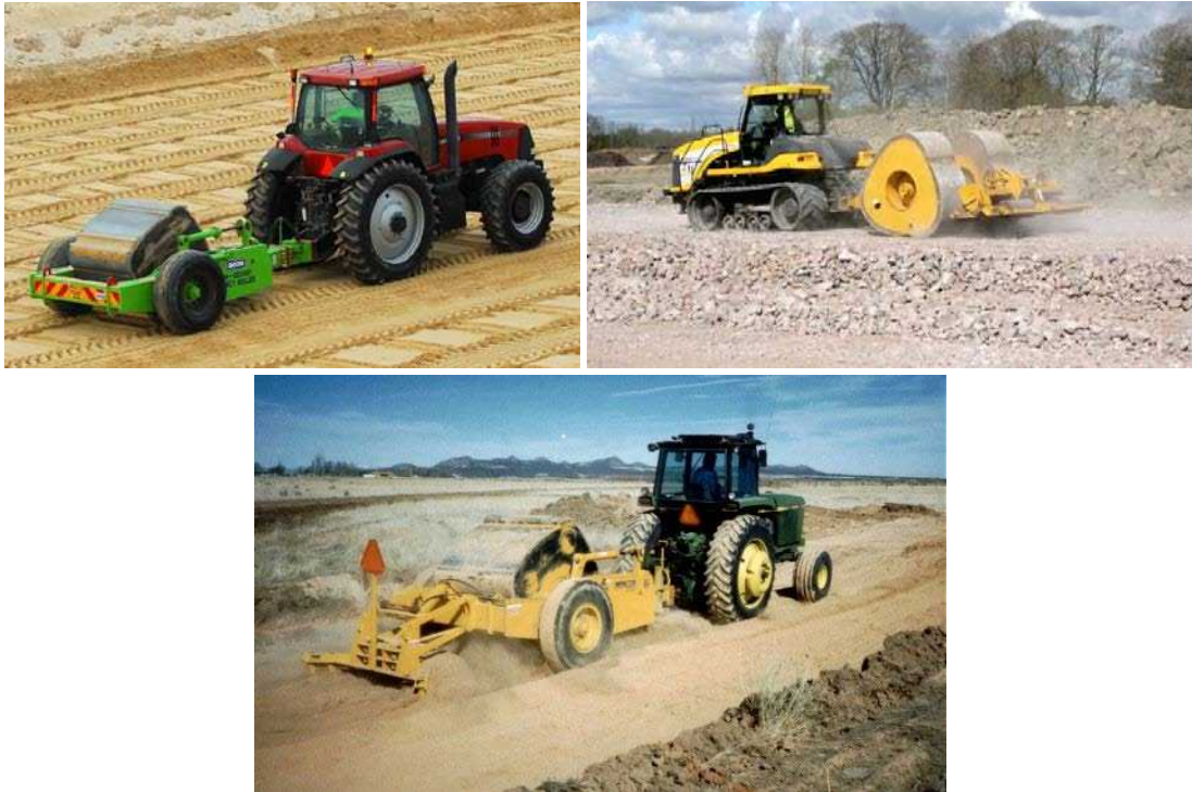
Figure 102. Broons (BH-1300) four-sided (“square”) impact roller towed using a four wheel drive heavy tractor (top left, Broons 2009); Landpac 25-kJ three-sided impact roller (top right, www.landpac.com/landpac%20apps%20and%20servs.html ) ; IRT’s Impactor 2000 “square” impact roller (bottom, www.impactor2000.com/soil.html )
