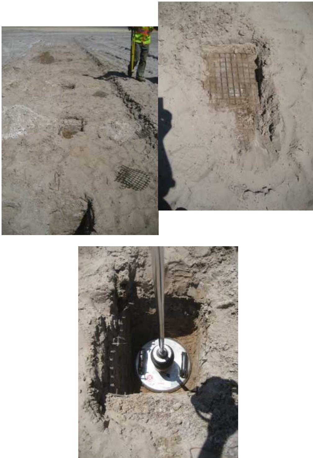
Figure 73. LWD testing in excavations at about 100 mm and 450 mm below surface – TB2
