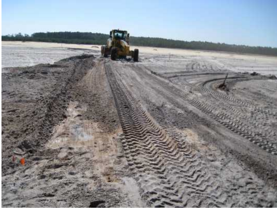
Figure 68. Loose lift leveling process – TB2
