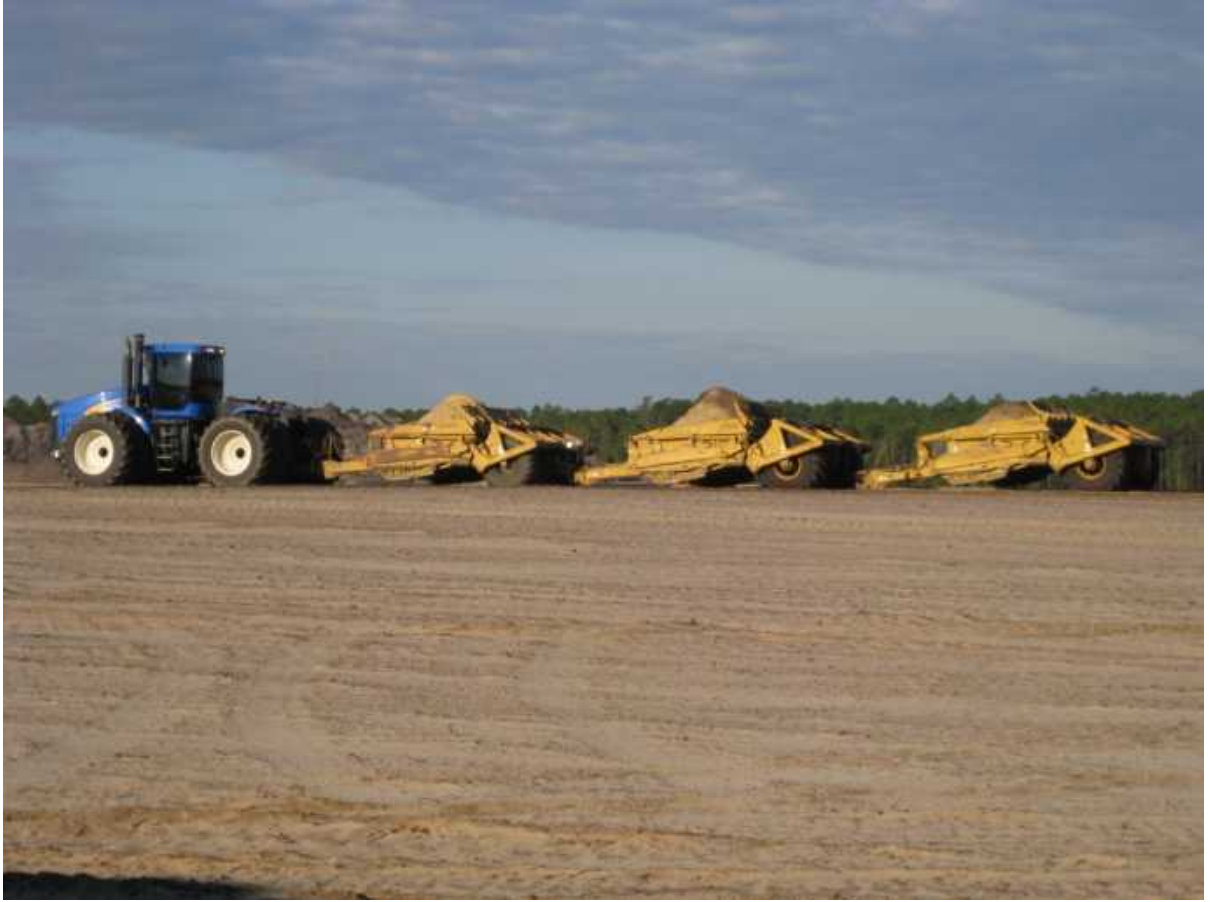
Figure 90. Pull behind scrapers used for hauling fill material and also for compaction on site
