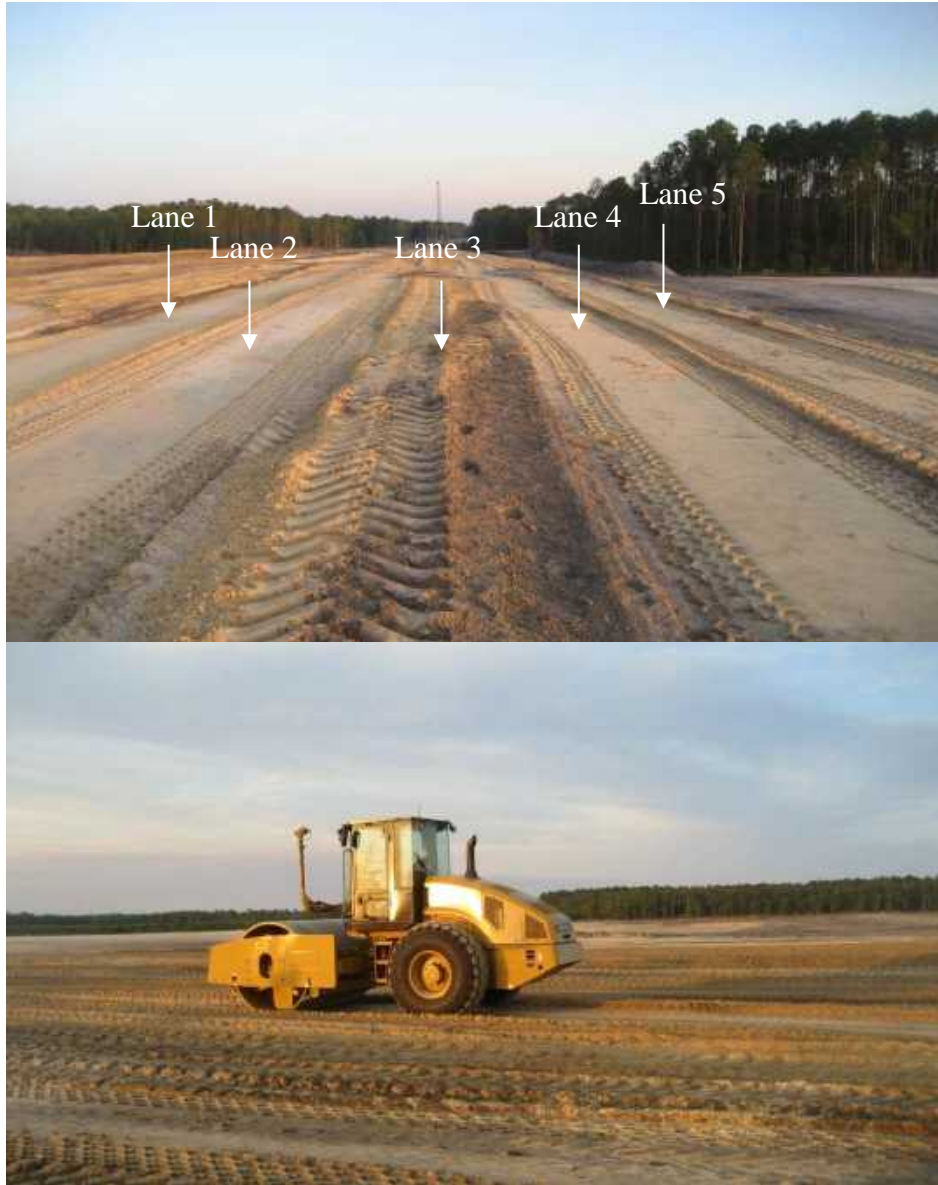
Figure 89. Pictures of production area test bed compaction (compaction on the test bed was achieved using contractors' equipment (see next picture); lanes 1, 2, 4, and 5 were mapped using the CS74 roller after compaction and lane 3 was not mapped but tested using DCP, LWD, and NG for comparison between mapped versus unmapped lanes) – TB3
