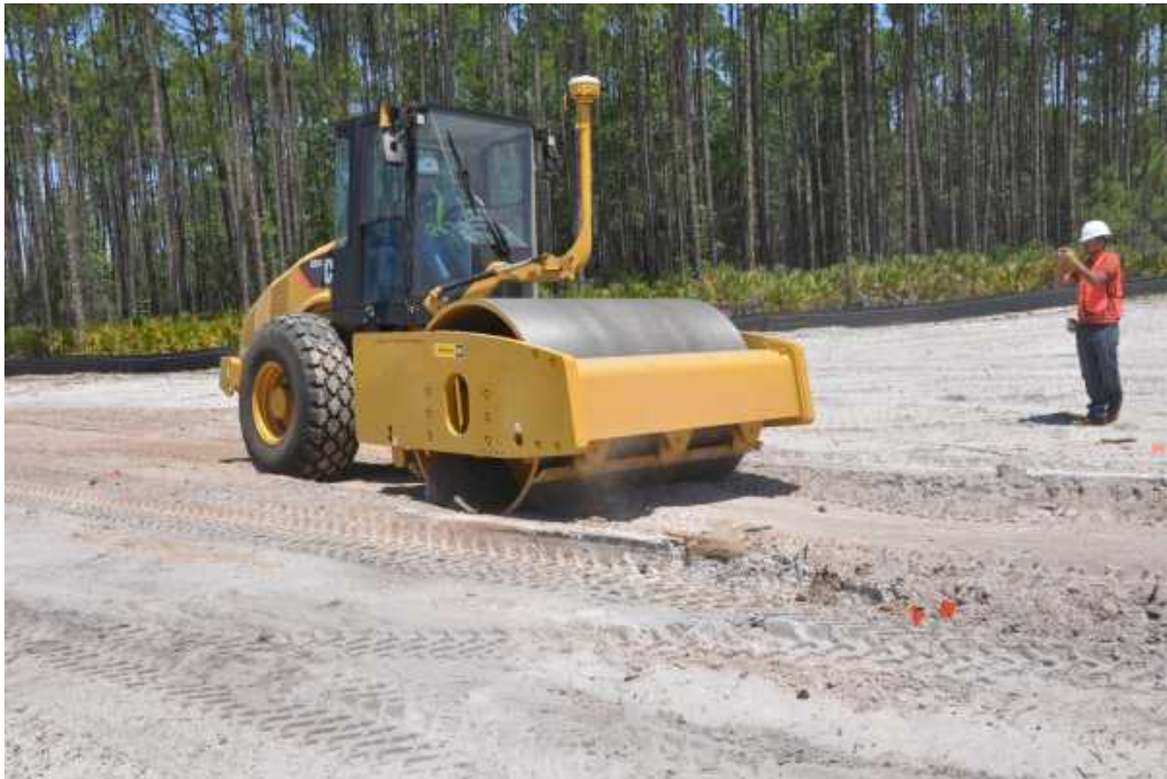
Figure 71. Compaction of test bed using CS74 vibratory smooth drum roller ( a = 1.80 mm) – TB2
