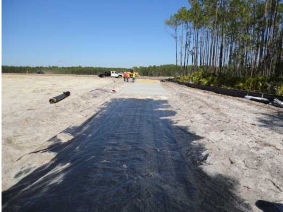
Figure 27. Woven fabric (PPWF) placed on the sand base layer – TB1
