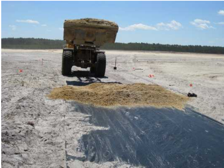
Figure 30. Fill layer 1 placement on PPWF section – TB1
