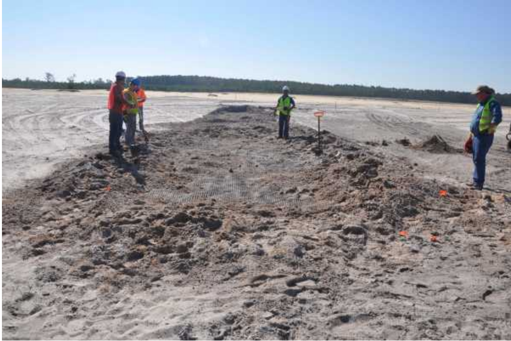
Figure 70. Fill placement (~100 mm thick) over BX geogrid – TB2
