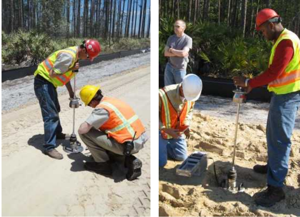
Figure 31. LWD testing on surface (left) and in excavation (right) – TB1
