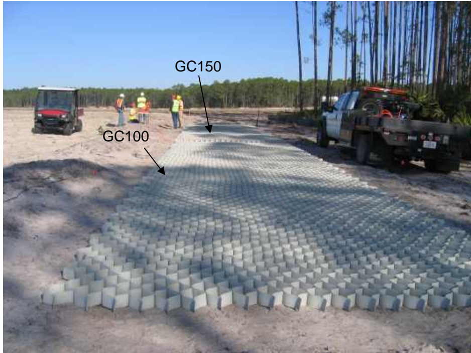
Figure 25. GC150 and GC100 installed on the sand base layer – TB1
