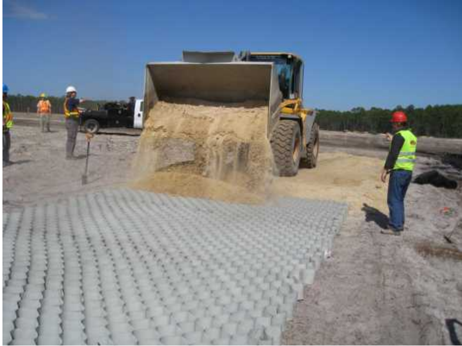
Figure 29. Fill layer 1 placement on GC150 section – TB1
