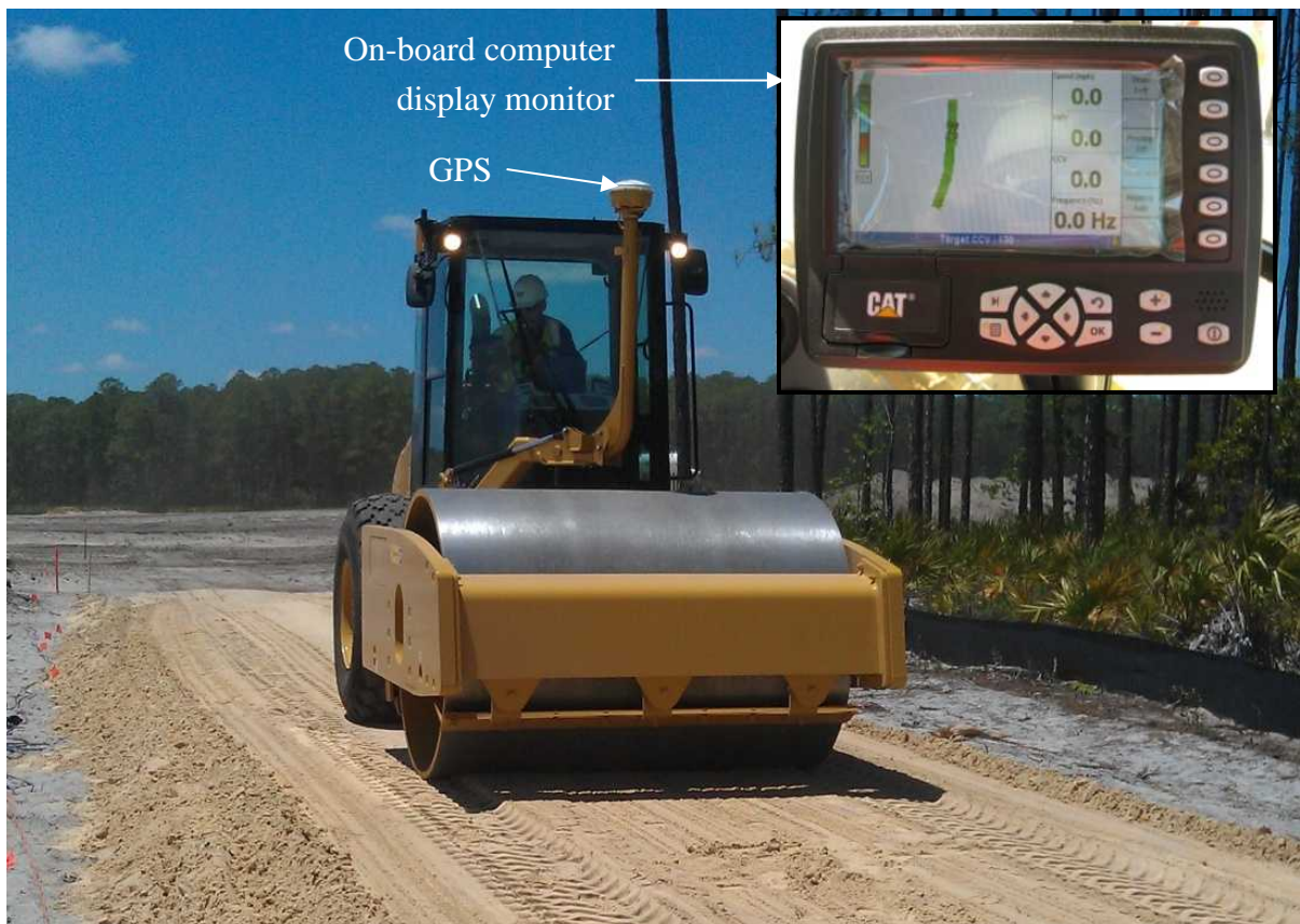
Figure 2. CS74 vibratory smooth drum roller with on-board computer display shown in the insert
