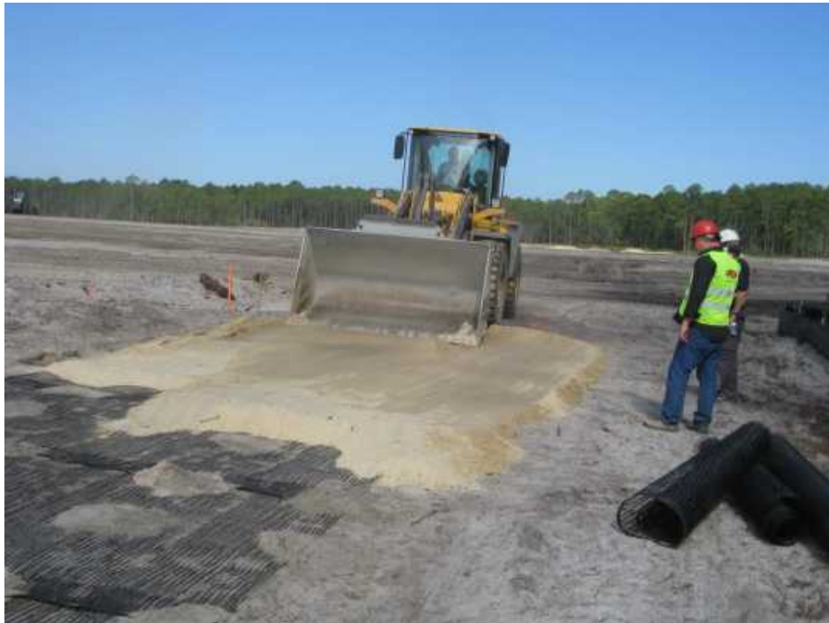
Figure 28. Fill layer 1 placement on BX geogrid section – TB1
