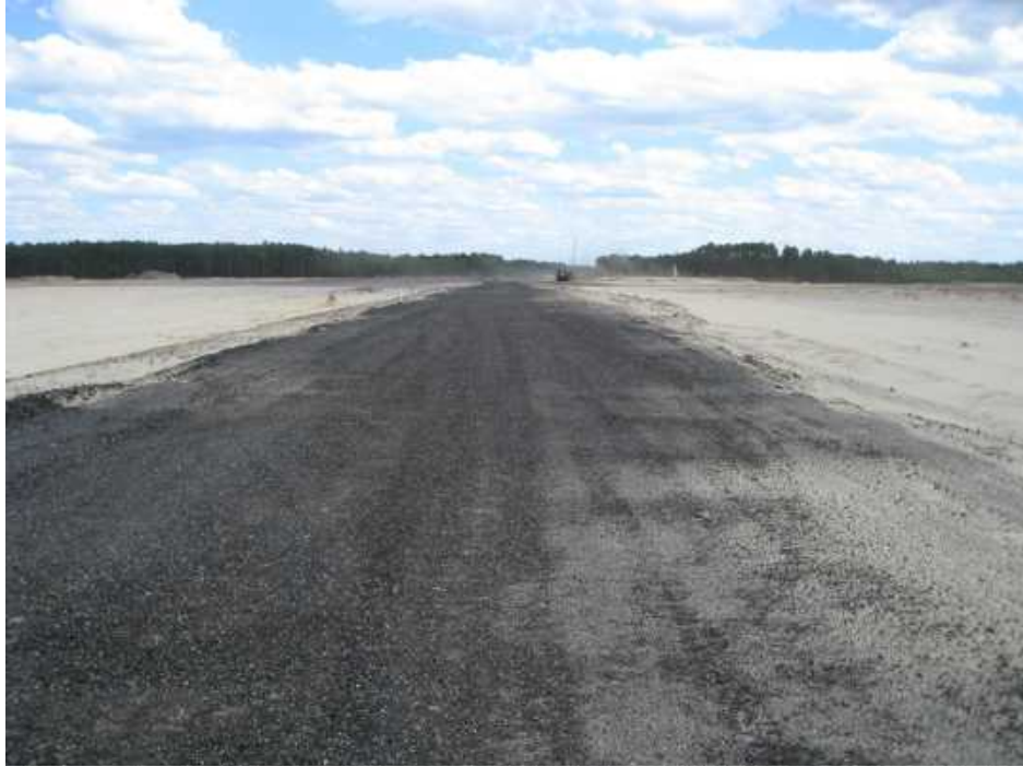
Figure 80. Picture of TB3 recycled asphalt pavement (RAP) surfacing on sand subgrade
