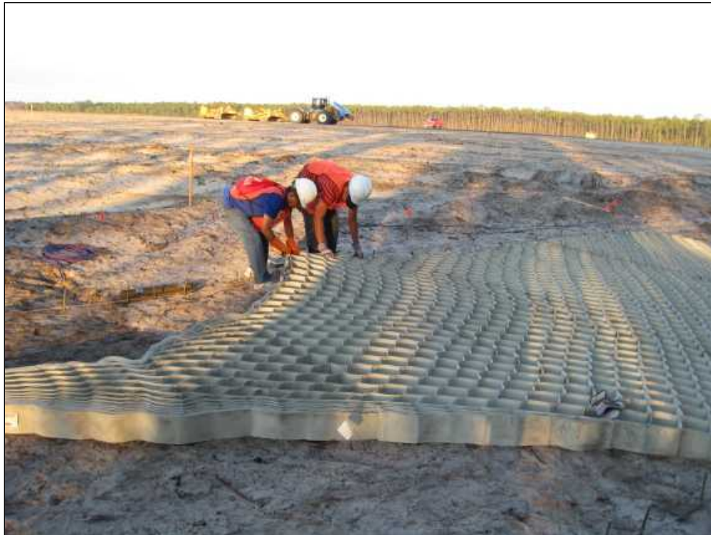
Figure 24. Stretching the geocells – TB1
