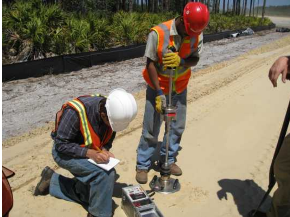
Figure 8. LWD testing using Zorn 300 mm diameter plate
