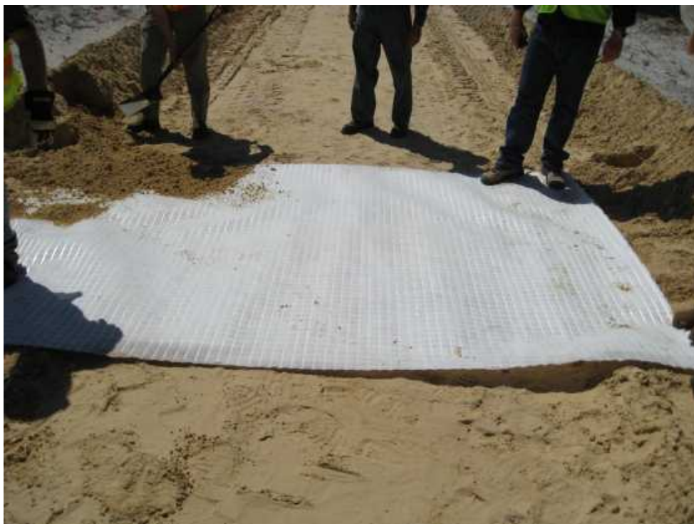
Figure 4. Pictures of C30 geogrid/nonwoven geotextile geocomposite used in this study
