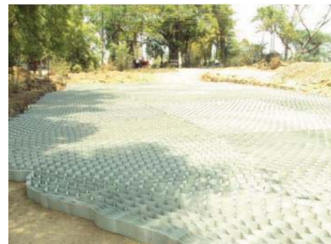
Fig. 3 Geocell layer spread over the road section
