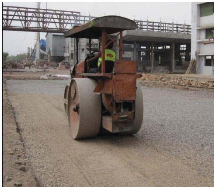
Fig. 5 Compaction by a vibro roller
