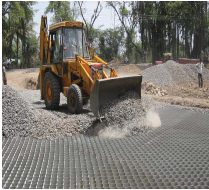
Fig. 4 Filling the geocell pockets
