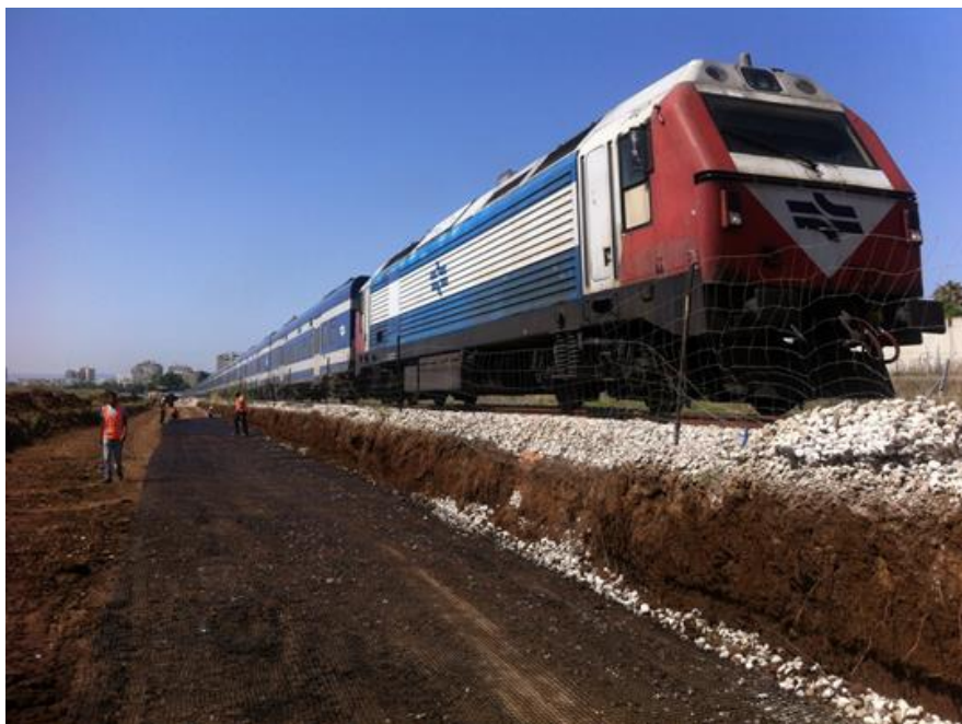
Figure 4. Keeping the Western track service live while constructing the adjacent new Eastern Track
