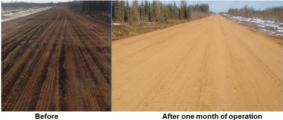
Figure 3. Driving condition on C-road before and after installation of Neoloy Geocell reinforcement
