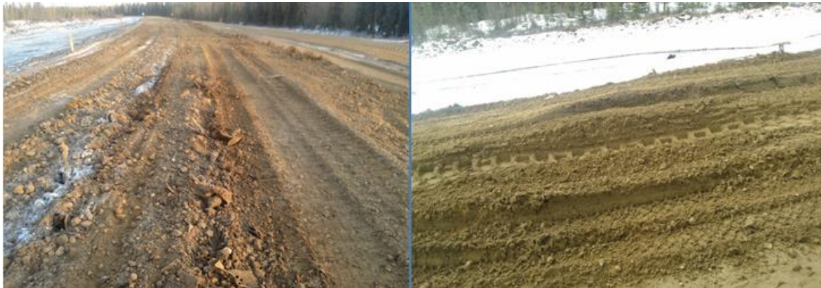
Figure 4. Failure after exceeding the design traffic at the J-Hook road
