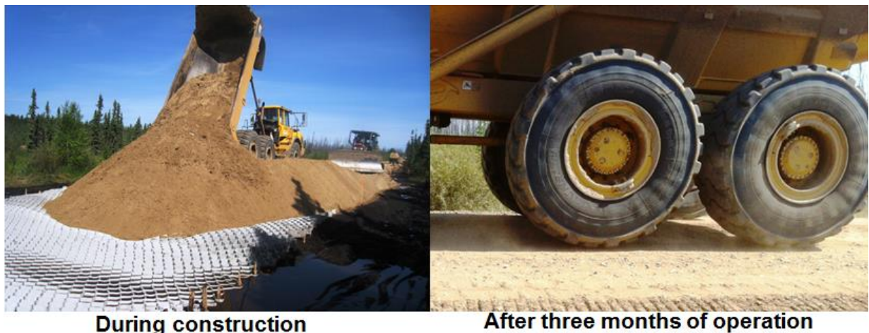
Figure 2. P-3 connector during construction and during the heavy traffic period
