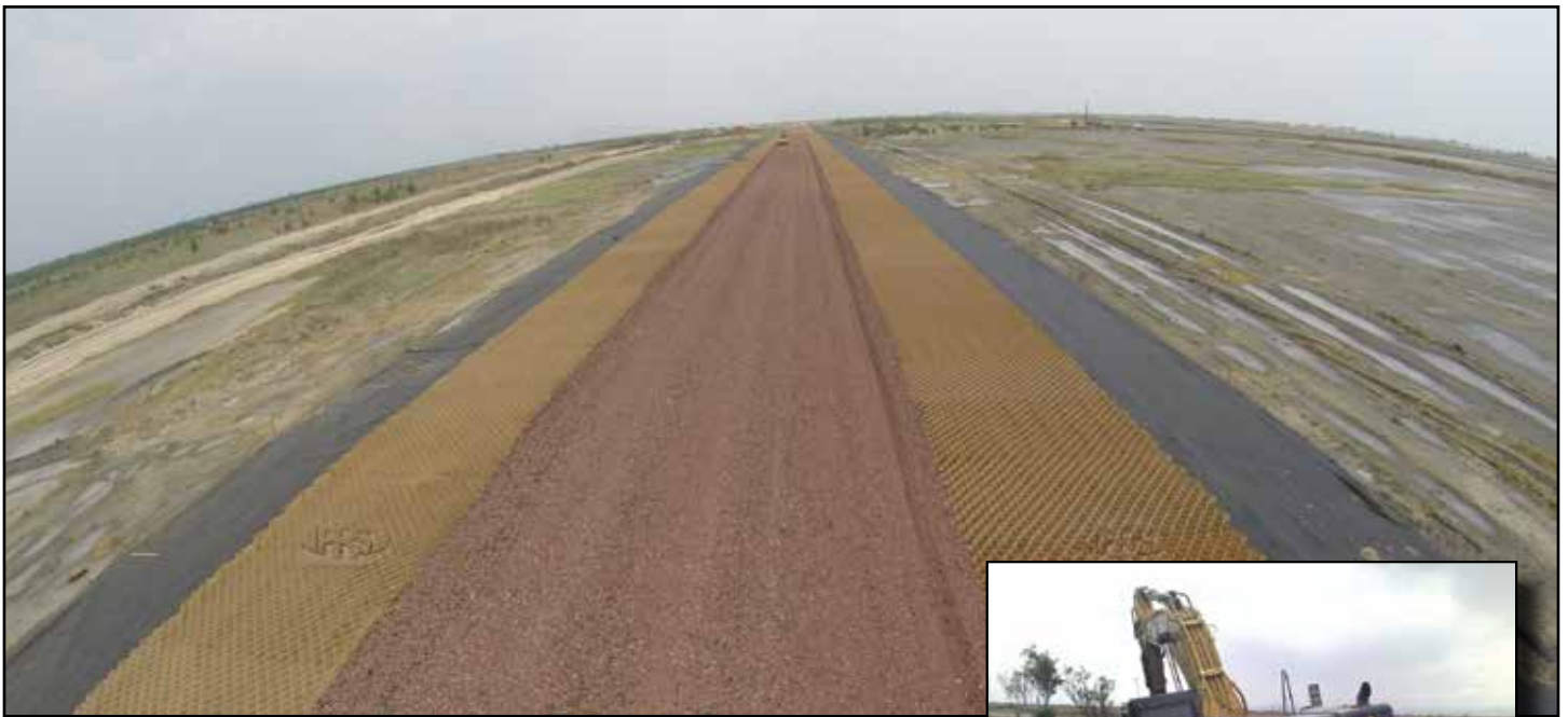
Above: Partially infilled NPA geocell road construction over clay mud swamp. Inset: Heavy construction machinery sinking in airport's soft clay mud (no NPA geocell reinforcement). Photo credits: Innovater
