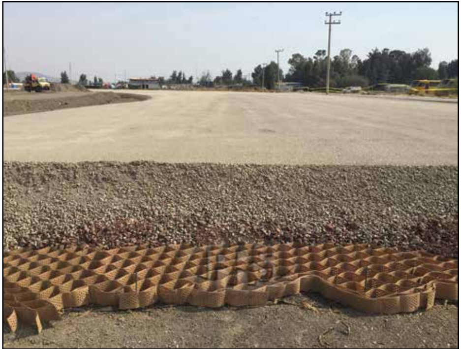
NPA geocells can reduce asphalt layer by 20% and structural layers by 50%.
