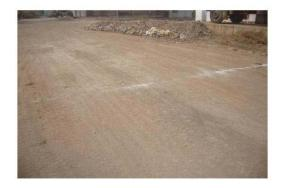
Fig. 7 Geocell reinforced pavement with uniform surface
