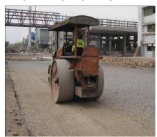
Fig. 5 Compaction by a vibro roller
