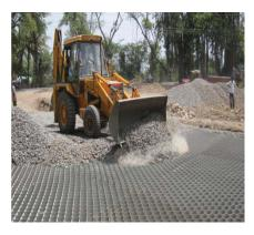
Fig. 4 Filling the geocell pockets
