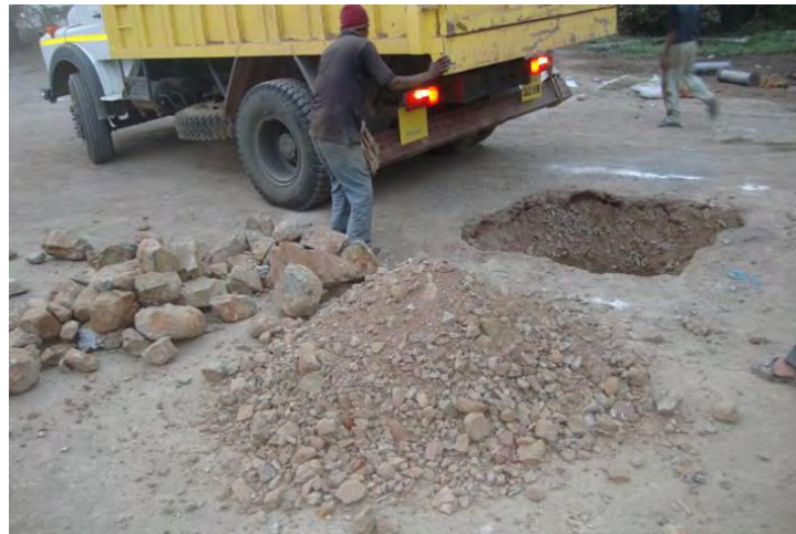
Figure 4. Bouldery size stones present at the subgrade level of unreinforced section
