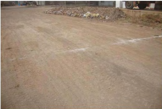
Figure 3. Neoweb reinforced road section showing level surface
