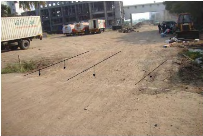
Figure 2. Unreinforced road section with severe surface depressions
