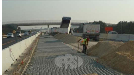
Figure 4. Installation of Neoweb on Highway 6
