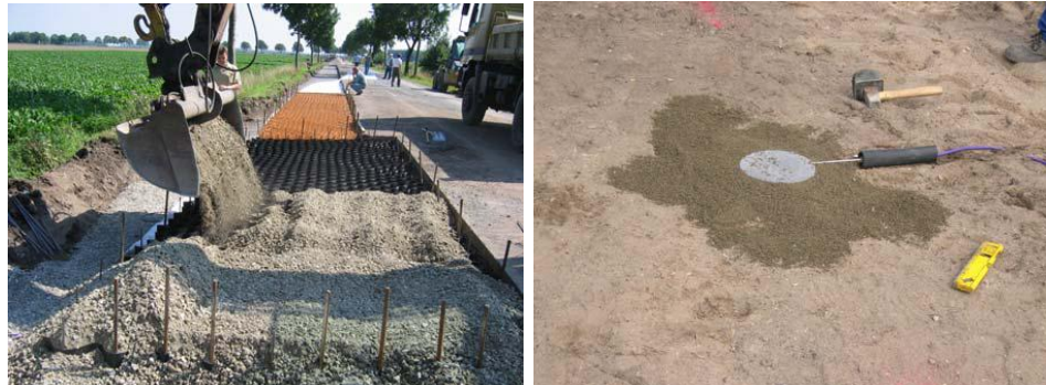
Figure 2: Installation and Infill of the Geocell (L), Earth Pressure Cells (R)
