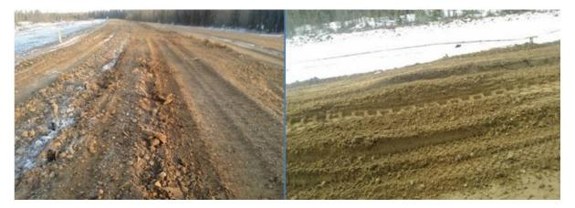
Figure 4. Failure after exceeding the design traffic at the J-Hook road
