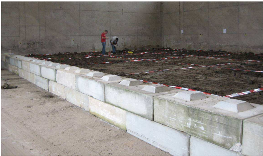
Figure 2 Overview of test site and marking of test sections 4x4 m 2
