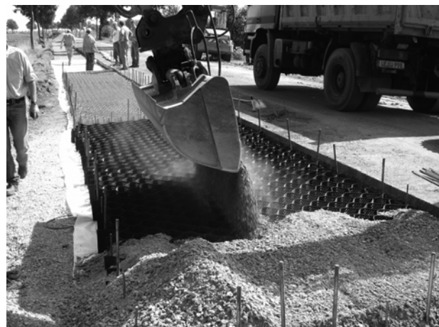
Fig. 4: installation of geocell layer directly beneath the asphalt surface
