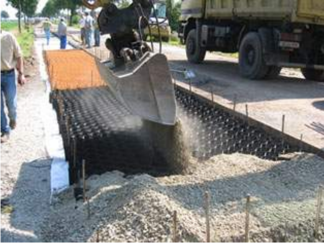
Figure 5: installation of geocell layer directly beneath the asphalt surface
