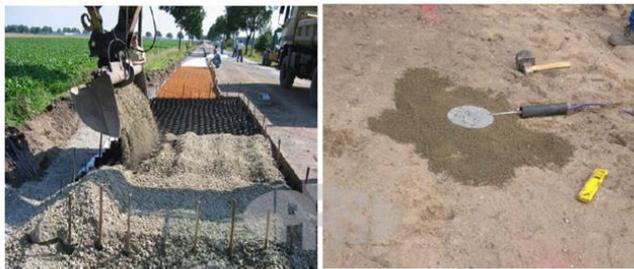
Installation and Infill of the Geocell (L), Earth Pressure Cells (R)
