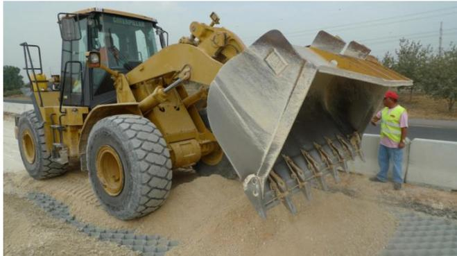
Figure 16. Installation of Neoweb in Cross Israel Highway 6
