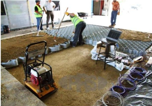
Figure 02: Installation of Neoweb and instrumentation in Accelerated Pavement Testing (APT) facility, Kansas
