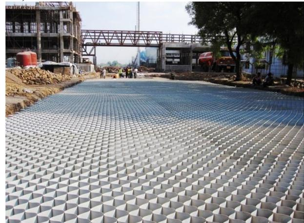
Figure 12. Neoweb installation of access road, Phaltan, India
